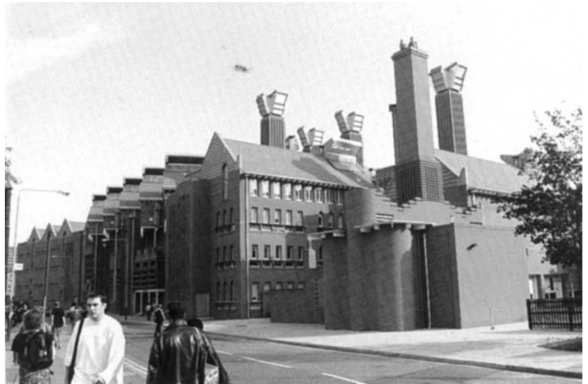
Figure 2.17 Queen's Building, School of Engineering and
